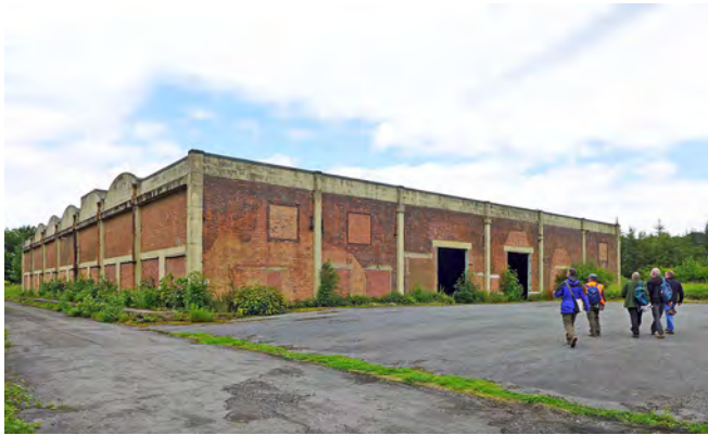
Sub Brit members head towards building P4. This Grade II listed building was intended to house plant for the production of Pyro mustard. As the threat of invasion receded the building wasn't used for production.
